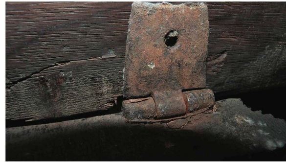
Fig. 17 Example of mortised knuckle hinge with flange out of mortise, Norwich.
